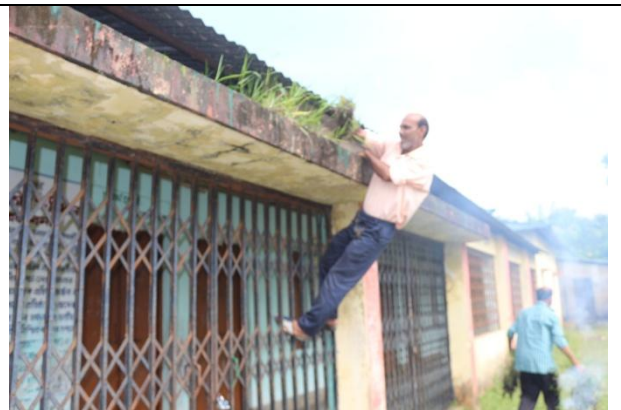
Cleaning the school roof
